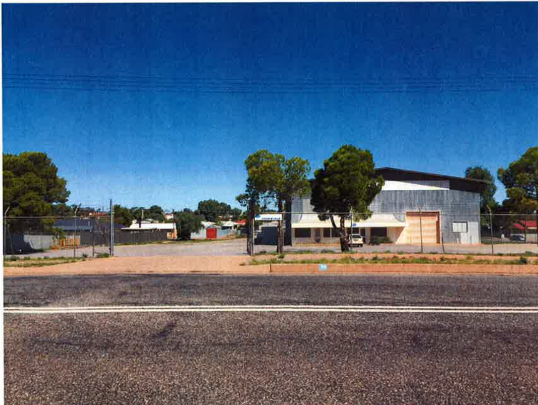
Photograph 1: Taken from Morgan Street, showing the subject site, with existing shed and carparking area.
